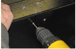
16. Enlarge the holes with a 3/8" drill bit for the nut inserts.
