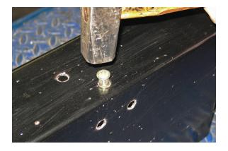
18. Place the supplied hex insert tool on top of the mounted nut inserts in the frame. Aligned with the insert, place a 1/4"-20 x 1-1/4" bolt and 1/4" washer into the nut insert.
