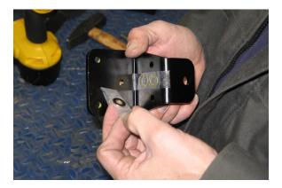
21. Place the bracket on top of the frame mounted nut inserts and fasten the top and bottom of the bracket with the 1/4"-20 x 1-1/4" bolts and 1/4" washers. Torque to 11 ft lbs.
