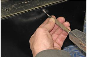
15. Use a 1/8" drill bit to drill pilot holes on all marks that have been punched.
